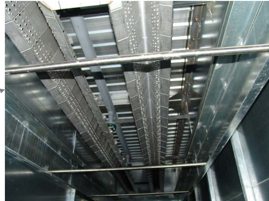
Burners Installed Inside Air Supply House
