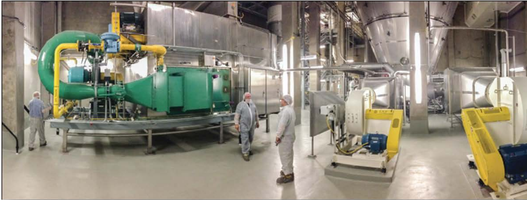
ER Heater Installation at Spray Drying Facility
